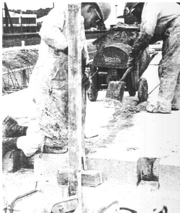
Fig. 4.3 -- Epoxy grouting of keyways in rapid transit bridge (courtesy Adhesives Engineering)
