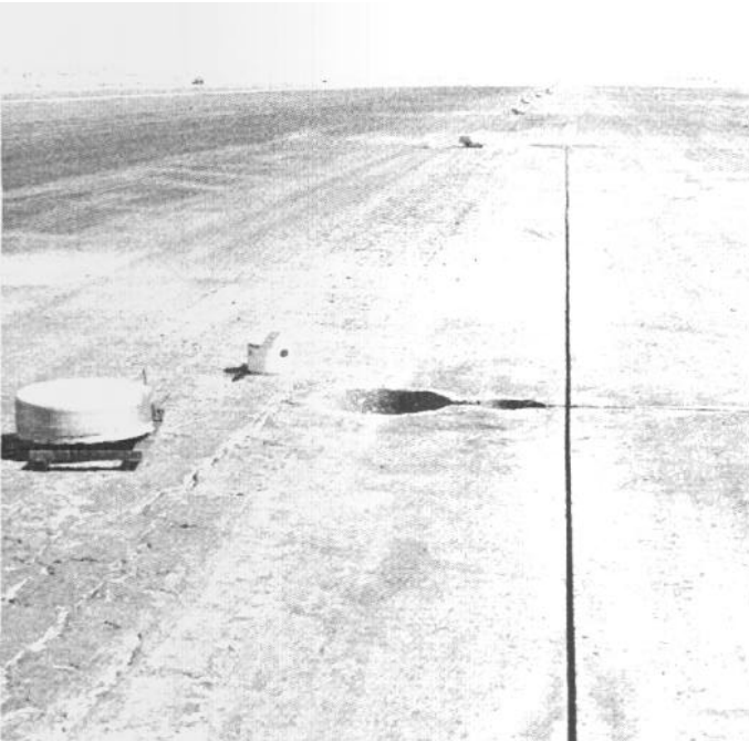
Fig. 7.6 -- Embedment of center line lighting in runway. Holes were cored, mixed epoxy poured therein and the light and junction boxes set and grouted (courtesy Adhesives Engineering)
