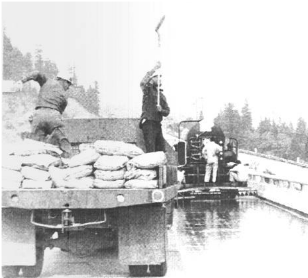
Fig. 7.3 -- Skid resistant calcined bauxite being applied by an automatic seeder for improved uniformity of coverage (courtesy Adhesives Engineering)
