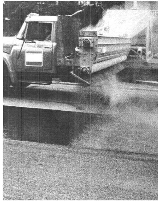
Fig. 7.3 -- Skid resistant calcined bauxite being applied by an automatic seeder for improved uniformity of coverage (courtesy Adhesives Engineering)
