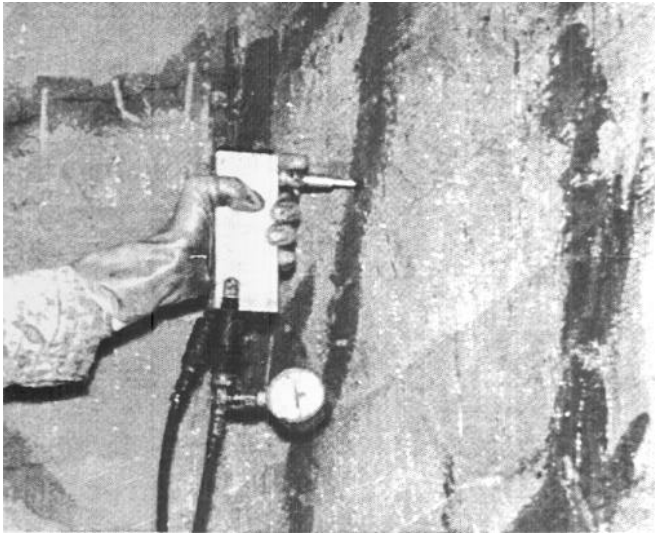
Fig. 6.4 -- A continuous mixing head gun being used for crack injection. Note that a thermoplastic surface seal was first applied, then through entry ports in the sealer the gun pumps the adhesive (courtesy Adhesives Engineering)
