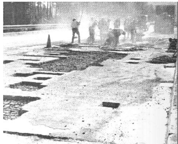
Fig. 5.1 -- Removal operation of all unsound concrete in bridge deck down to top steel. Repair was made by bonding the fresh high early strength concrete patch to the old concrete using an epoxy adhesive at the interface (courtesy Adhesives Engineering)
