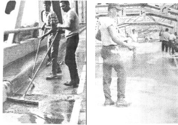
Fig. 7.2 -- Squeegee and roll on application of seal coat followed by skid resistant layer spread by a hand seeder (courtesy Sika Chemical Corp.)
