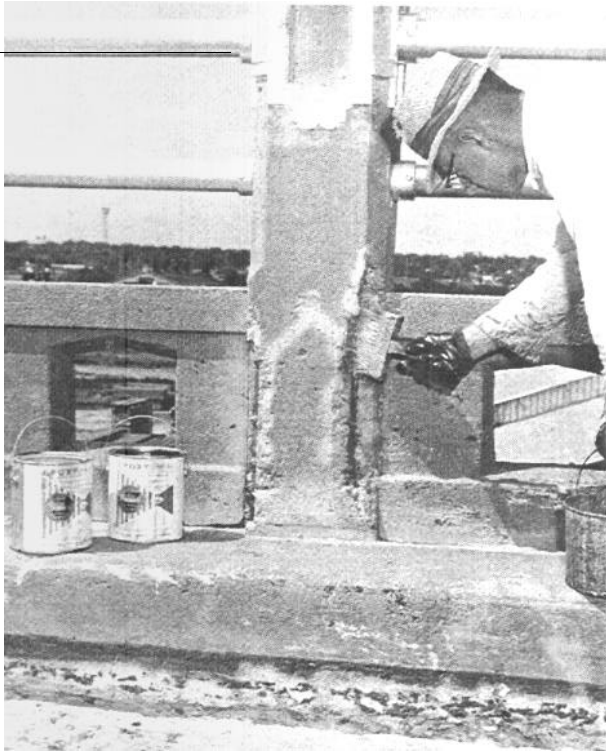
Fig. 4.4 -- Repair of a concrete bridge railing upright (courtesy Protex Industries)
