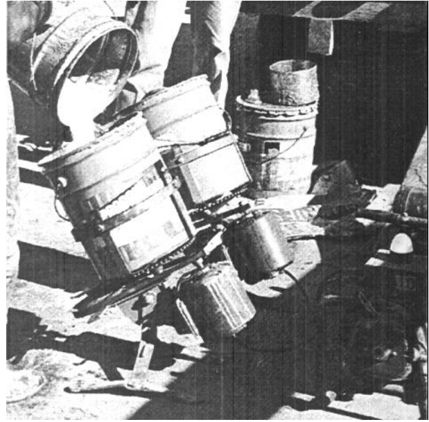
Fig. 6.2 -- Rotating bucket mixing of epoxy compounds (courtesy Protex Industries)
