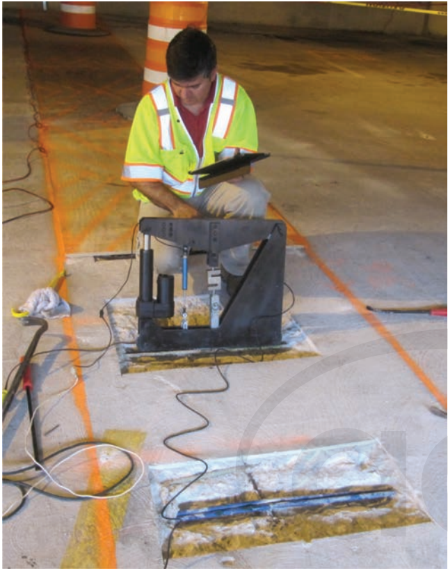
Fig. 5.4.3.2b—In-place tension testing of unbonded tendon.
