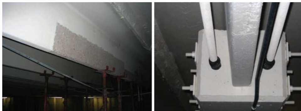
Fig. 7.4.1b—External post-tensioning of precast tee member prior to repair with shoring in place (left), and after reinforcement is placed and encased at the center of the tee stem (right).
