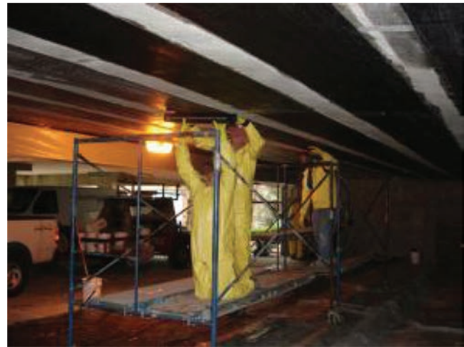
Fig. 7.3.2c—FRP reinforcement.
