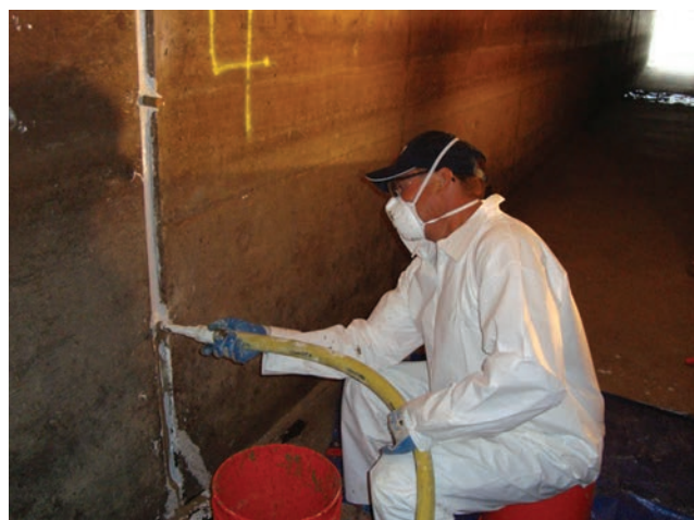
Fig. 5.2.2.1—Chemical grouting.
