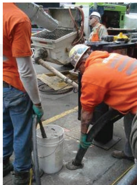
Fig. 5.2.2.2—Cement grouting.
