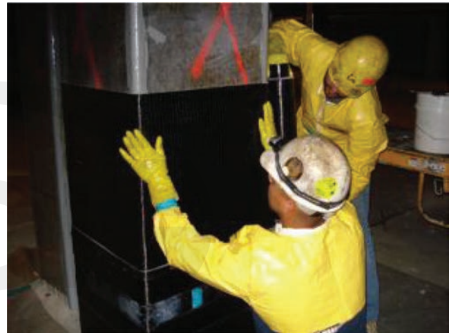
Fig. 7.3.2d—FRP reinforcement.
