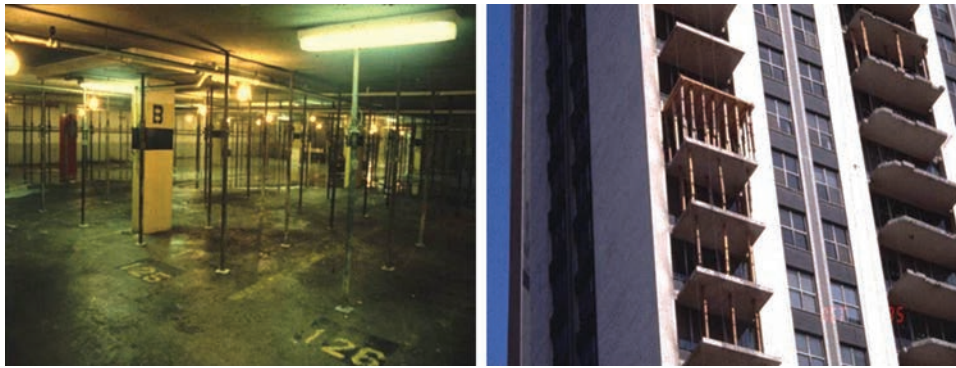
Fig. 3.2.2a—Temporary shoring parking garage floor (left) and balcony slabs (right).
