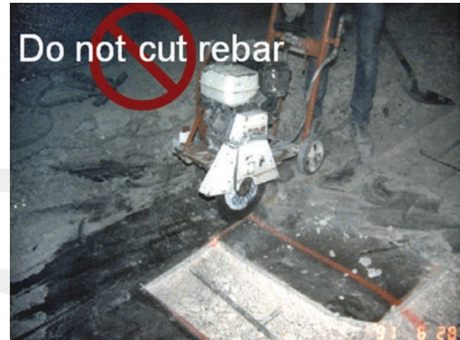
Fig. 3.2.2b—Saw cutting perimeter of repair area.
