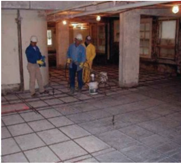
Fig. 5.3.9—Application of bonding material before overlay application.
