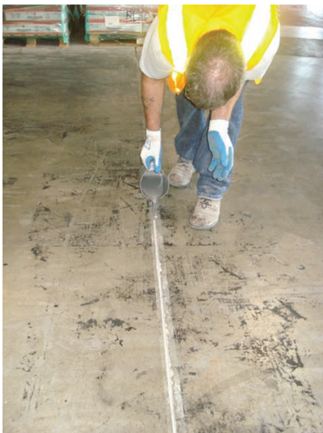
Fig. 5.2.1.2—Horizontal gravity feed of crack.
