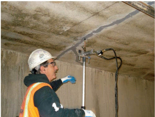
Fig. 5.2.1—Overhead epoxy injection of crack.
