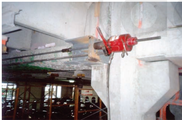
Fig. 7.4.1a—External post-tensioning of prestressed girder.
