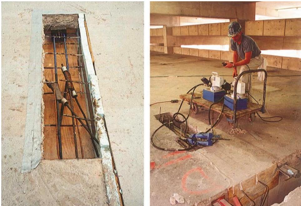
Fig. 5.4.3.2c—Tendon splices in place (left) and being restressed (right).
