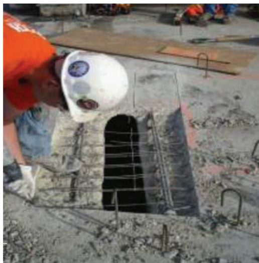
Fig. 5.3.1—Horizontal repair at full depth.
