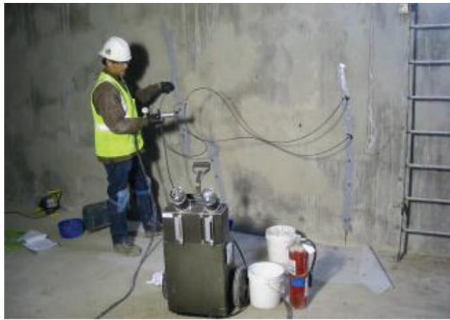
Fig. 7.2.1—Epoxy injection of crack in wall.
