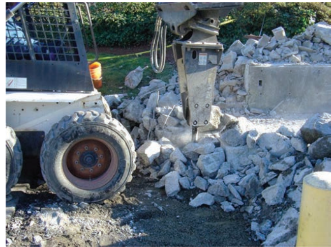
Fig. 3.2.4.2.2—Boom-mounted breaker.
