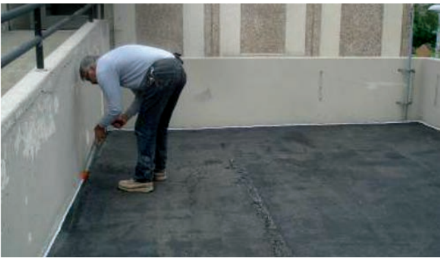
Fig. 5.2.3—Sealant application.
