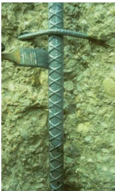
Fig. 5.4.2.3—Coating reinforcing steel.
