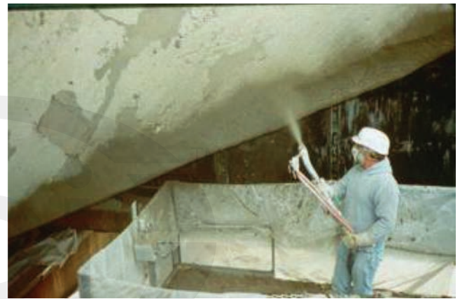
Fig. 5.3.5—Shotcrete method.
