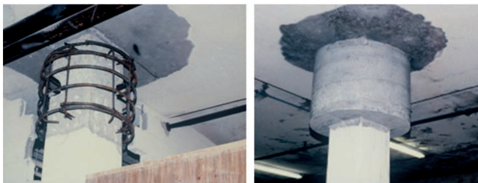
Fig. 7.5.1—Collar around top of column – reinforcement in place (left) and after concrete has been cast (right).
