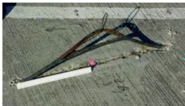
Fig. 5.4.3.2a—Failure of unbonded tendon.
