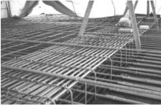
Fig. 2.3—GFRP bars used in a winery in British Columbia in 1998.
